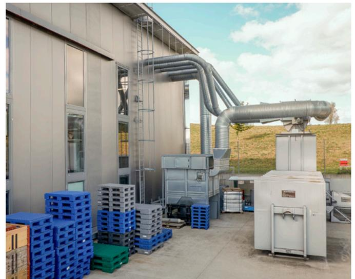
The suction plant in the BOBST Competence Center operates with an air volume flow of 24,000 cubic metres an hour.
