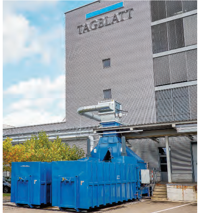
For economical, technical and logistical reasons, NZZ Media Services AG chose a double container compaction system.
